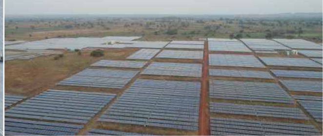
11.2 MW Solar PV Power Plant with Single Axis Tracking System, in Vikarabad, Telangana
