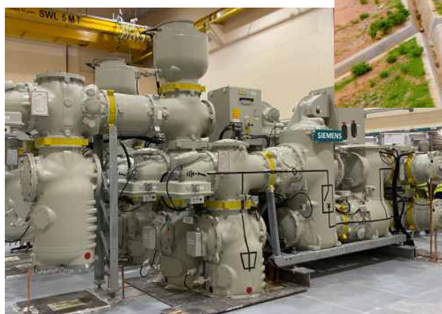
132 kV Gas Insulated Substation at Dubai, UAE
